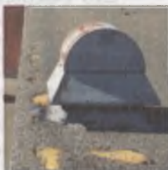
Deteriorating Foam Roof
