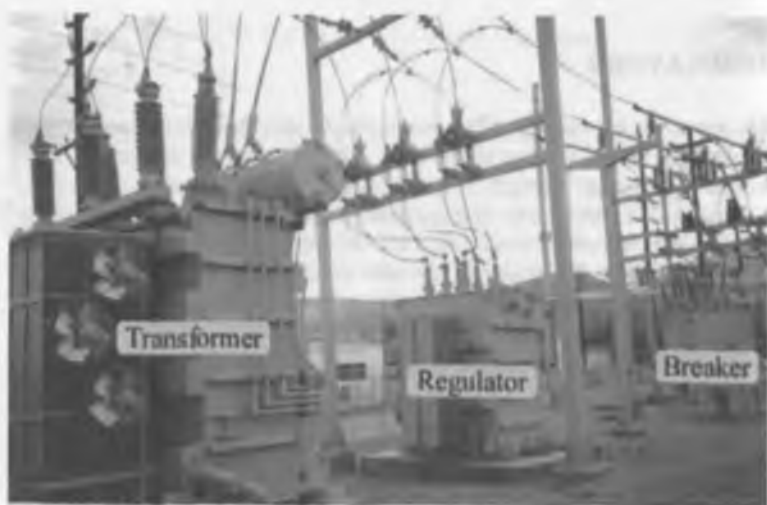
Figure 4-16. Three-phase regulator.
