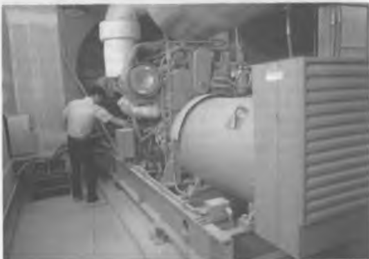
Figure 6-21. Emergency generator. Source: Photovault.
