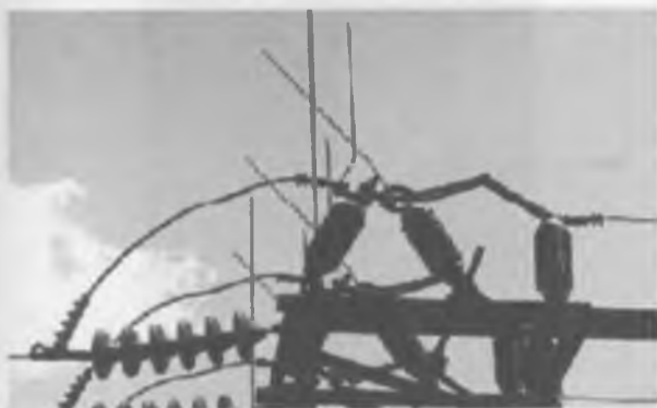
Figure 4-34. Arcing rods.
