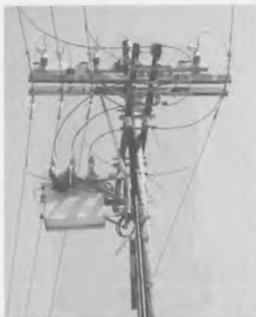
Figure 4-30. Distribution line recloser. Courtesy of Alliant Energy.
