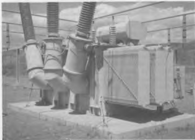
Figure 4-41. Reactor.
