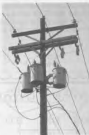
Figure 5-18. Three-phase transformer bank.
