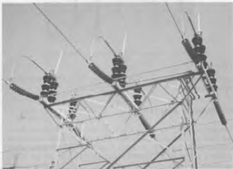
Figure 4-32. Vertical-break switch. Courtesy of Alliant Energy.
