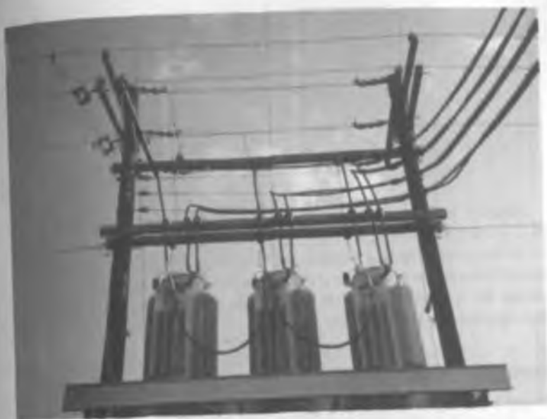
Figure 4-3. Transformer bank.
