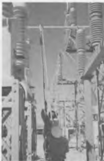
Figure 10-8. Live maintenance on transmission lines.
