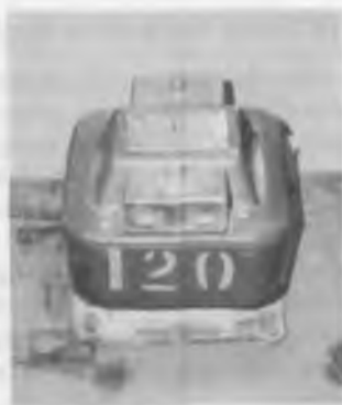
Figure 4-13. Low-voltage PT. Courtesy Alliant Energy.
