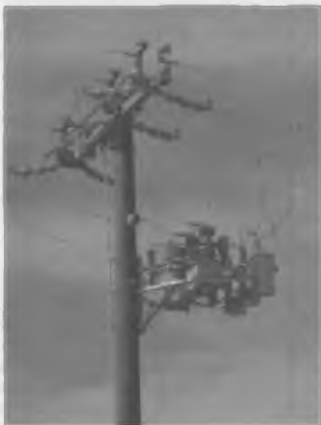
Figure 6-11. Overhead primary metering.
