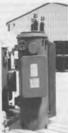
Figure 4-17. Single-phase regulator. Courtesy Alliant Energy.
