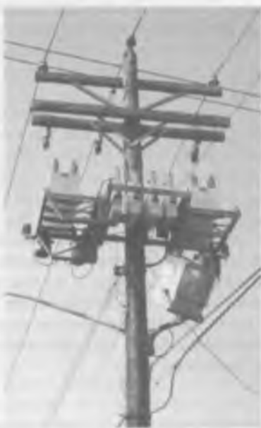
Figure 4-40. Distribution capacitor bank.
