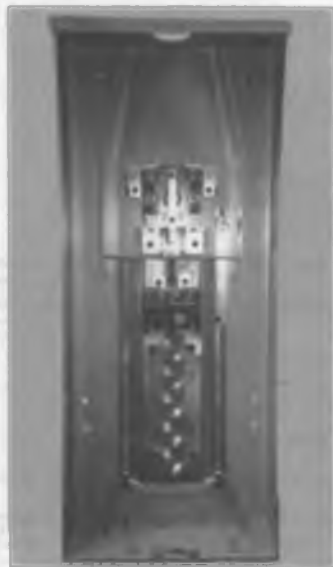
Figure 6-14. Breaker cover removed.
