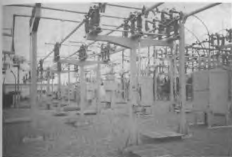
Figure 4-38. Examples of a typical electrical bus.
