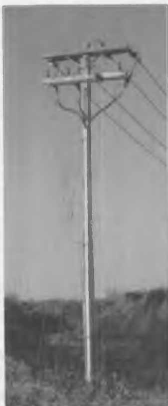
Figure 5-27. Dip pole.
