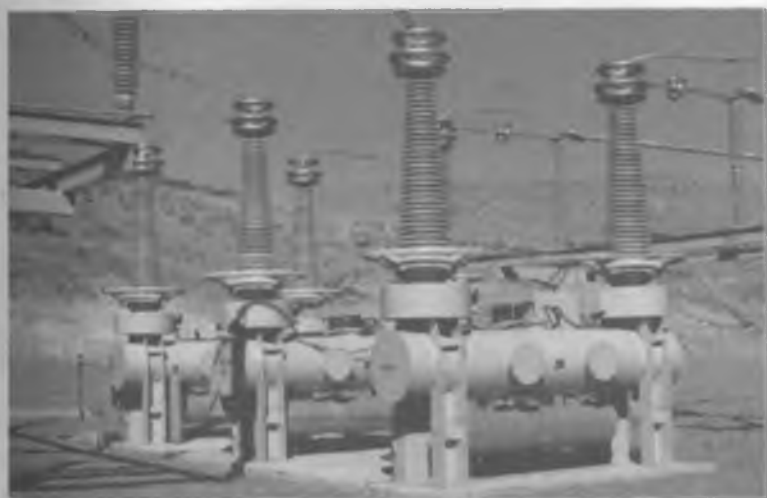
Figure 4-26. 345 kV Gas breaker.
