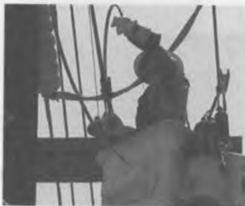
Figure 10-11. Live maintenance distribution. Courtesy of Alliant Energy.
