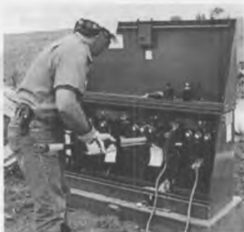
Figure 5-29. Load-break connections. Courtesy of Alliant Energy.
