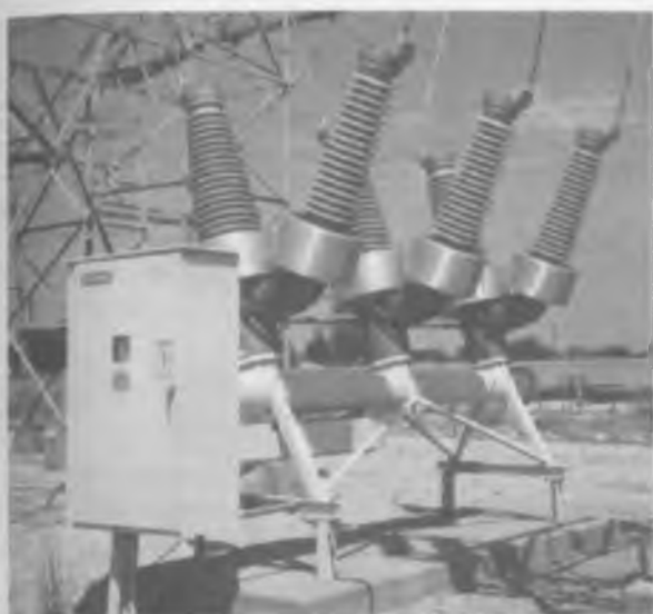
Figure 4-25. Gas circuit breaker.
