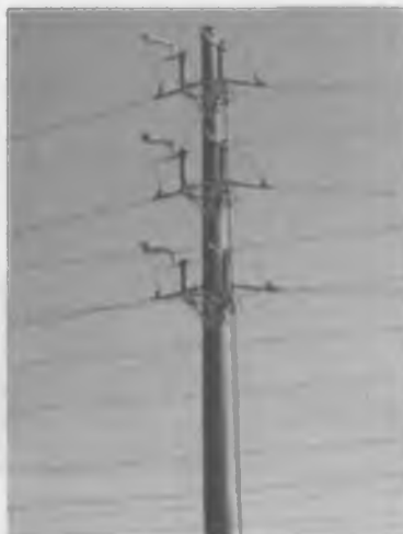
Figure 4-35. Line switch.
