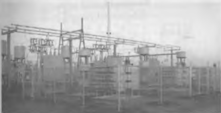
Figure 4-42. Static VAR compensator. Courtesy of Jeff Selman.
