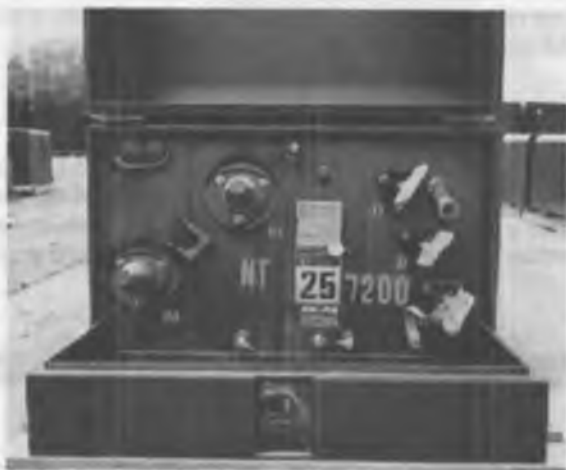
Figure 5-34. Switching transformer. Courtesy of Alliant Energy.
