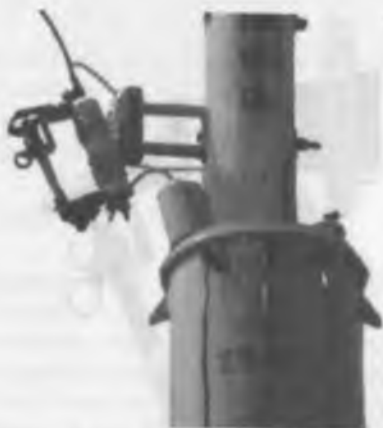
Figure 5.24. Distribution fuses.
