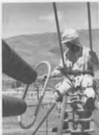
Figure 10-9. Bare-hand, live-line maintenance.
