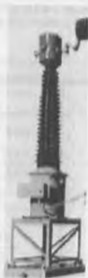
Figure 4-11. External high-voltage CT.
