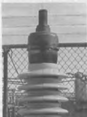
Figure 4-7. Bushing oil level gauge.
