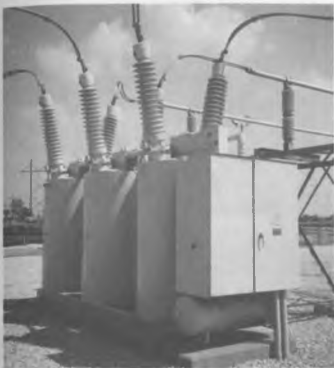
Figure 4-23. Oil circuit breaker.
