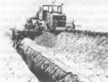
12.2-rasm. M3Y-2 mashinasining ishlash jarayoni.
