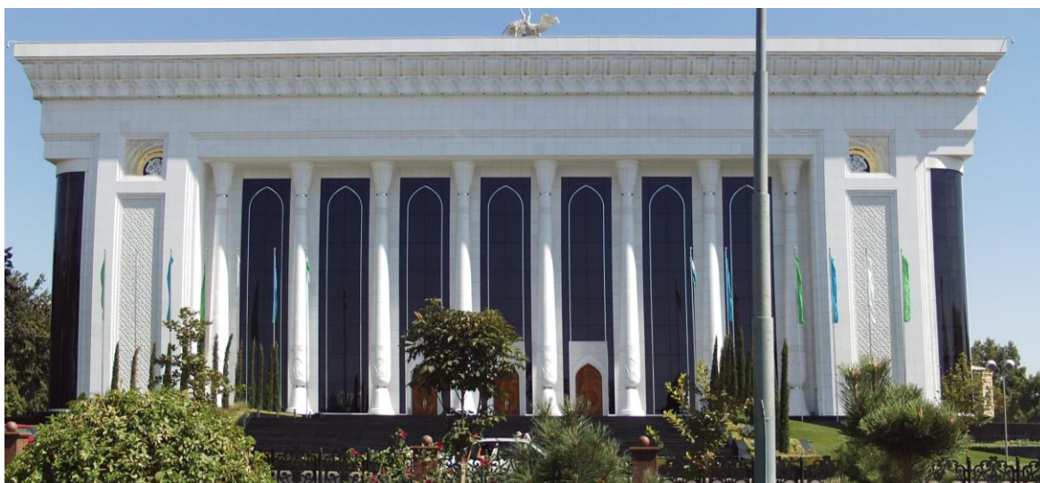
2.19-rasm. Marmarni zamonaviy binolarda (Toshkentdagi Forumlar zalining bosh fasadi) pardo materiali sifatida ishlatilishiga doir misol
