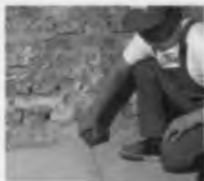
14.13-a rasm. Asosga pardevorning loyiha holatini belgilash.
