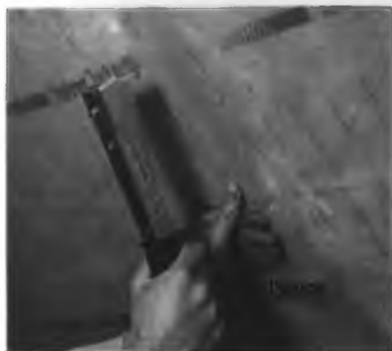
7.6-rasm. Stepler yordamida stropilaga nisbatan ko'ndalang ravishda plyonkani mahkamlash.
