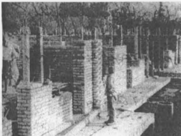
13.18-rasm. Temirbeton o'zakli g'isht devorning ko'rinishi
