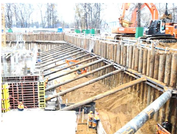
6.17-rasm. Tirgakli mustahkamlagichda mustahkamlangan kotlovan devorlari
