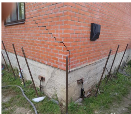
4.13-rasm. Grunt zaminining mustahkamlanmagan (a) va mustahkamlangan sharoitidagi binoning holati
