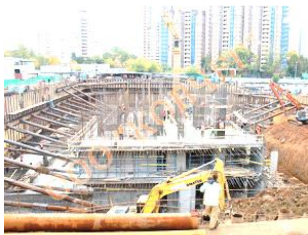
6.17-rasm. Tirgakli mustahkamlagichda mustahkamlangan kotlovan devorlari
