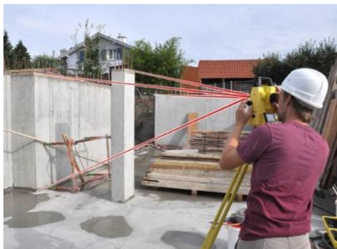
3.5-rasm. Leica Flexline TS06 plus (EGL) taximetri. Taximetp Leica bilan ishlash jarayoni
