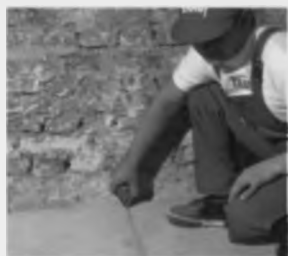
14.13-a rasm. Asosga pardevorning loyiha holatini belgilash.
