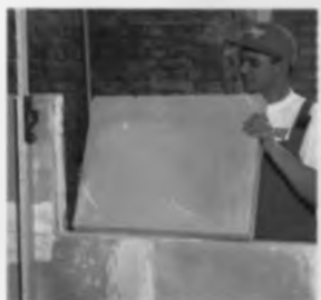
14.13-h rasm. Plitalarni terish choklarini ma'lum siljitish bilan amalga oshirish.
