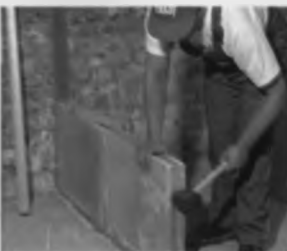
14.13-f rasm. Birinchi qator plitalari pravilo va shayton yordamida terish.
