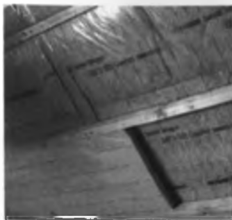
7.6-rasm. Stepler yordamida stropilaga nisbatan ko'ndalang ravishda plyonkani mahkamlash.
