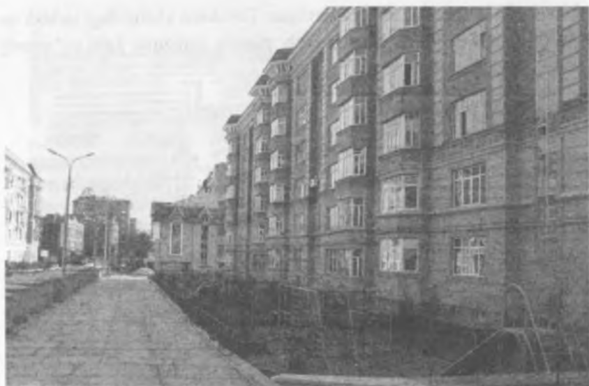
6.6-rasm. Toshkent shahridagi 6 qavatli zamonaviy turar-joy binosi
