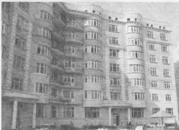
6.4-rasm Toshkent shahridagi 7 qavatli zamonaviy turar-joy binosi
