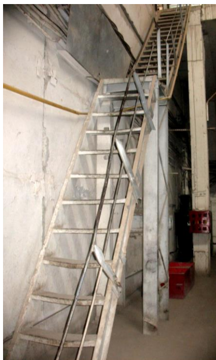
16.8-rasm. Tetiva va marshdan tashkil topgan metal zinapoyaning “Buxoroenergomarkaz” sexida qo‘llanilishi
