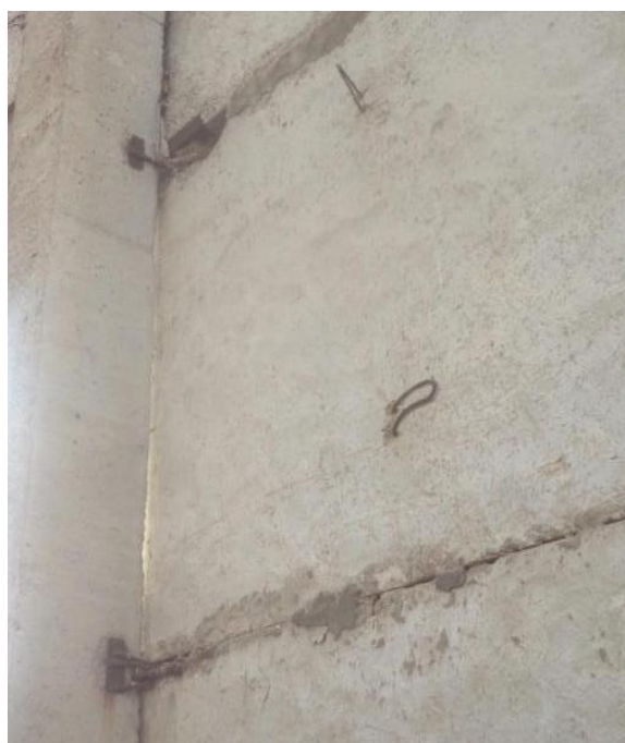
11.14-rasm. Sanoat binosining tashqi devor panellarini ustunlarga sharnirli mahkamlanishi
