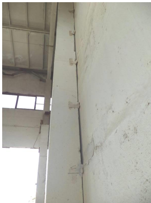
11.13-rasm. Sanoat binosining tashqi devor panellarini ustunlarga sharnirli mahkamlanishi
