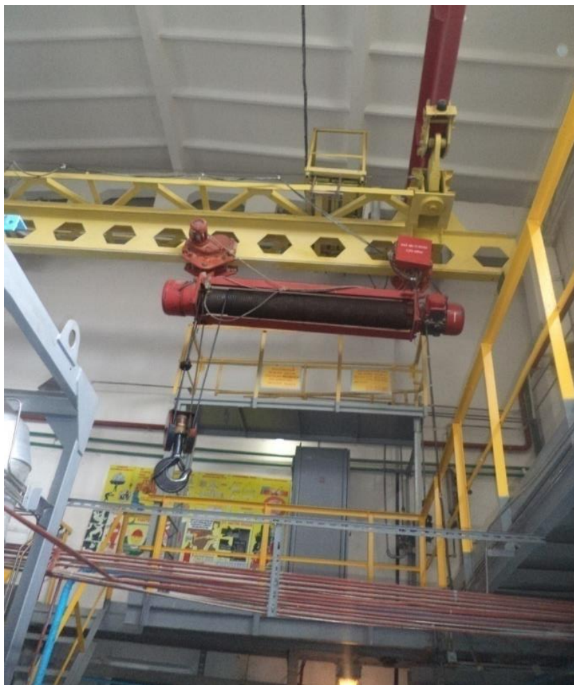
1.23-rasm. BNPZ kompressor stansiyasining kranli binosi
