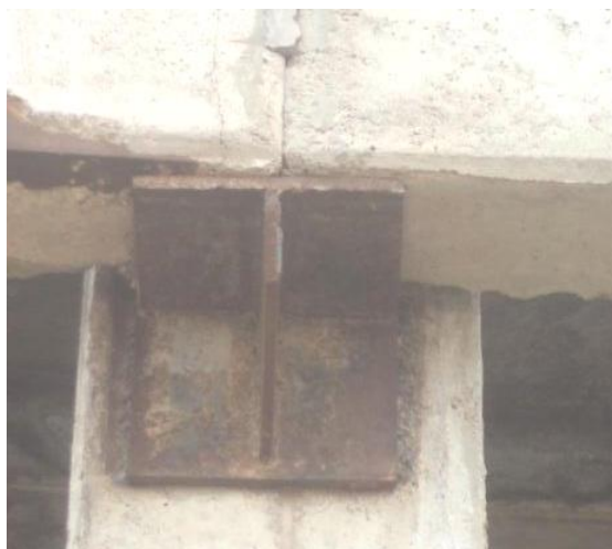
11.15-rasm. Sanoat binosining tashqi devor panellarini metall dan ishlanib, ustunga payvandlangan maxsus stulchaga mindirilishi
