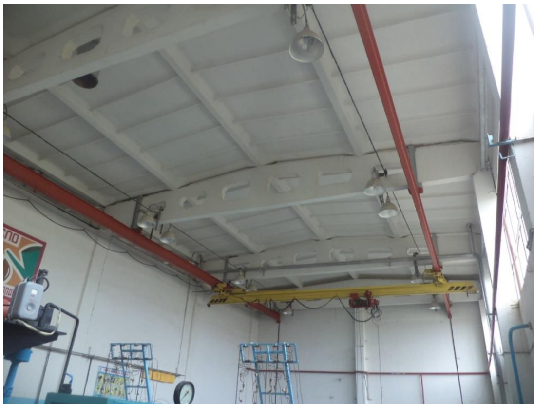
1.22-rasm. BNPZ kompressor stansiyasining kranli binosi
