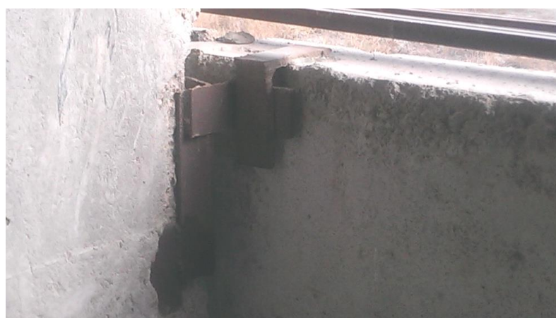
11.17-rasm. Sanoat binosining tashqi devor panellarini ustunlarga sharnirli mahkamlanishi
