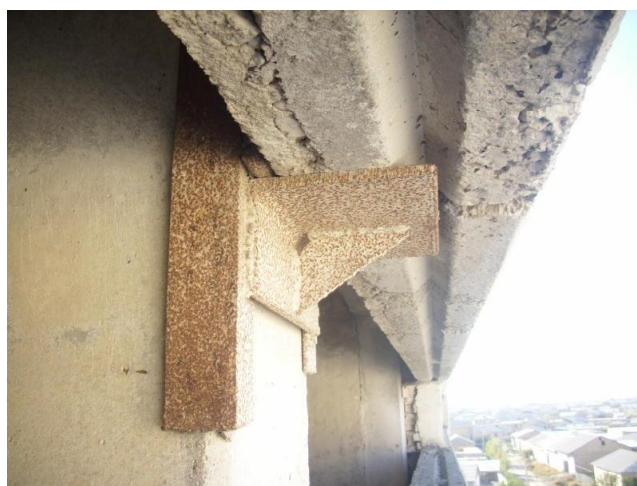
11.16-rasm. Sanoat binosining tashqi devor panellarini metall dan ishlanib, ustunga payvandlangan maxsus stulchaga mindirilishi
