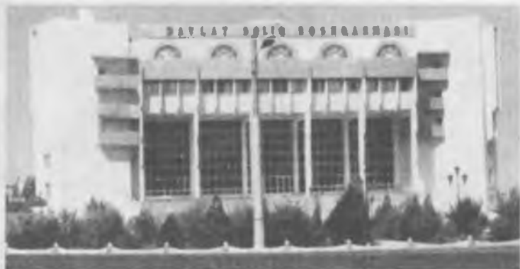
13.87-rasm. Urganch shahridagi soliq inspeksiya binosining ko'cha tomondagi fasadi
