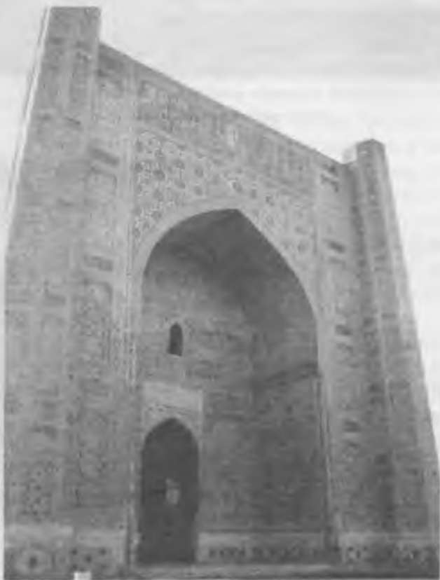
9.10-rasm. Masjid peshtoqining restavratsiyadan keyingi holati
