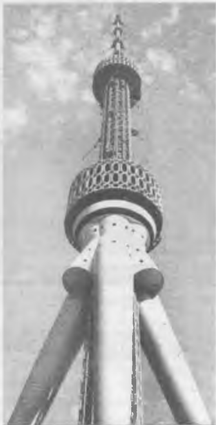
12.13-rasm. Toshkent shahridagi teleminora (1978–1985-yillar)
