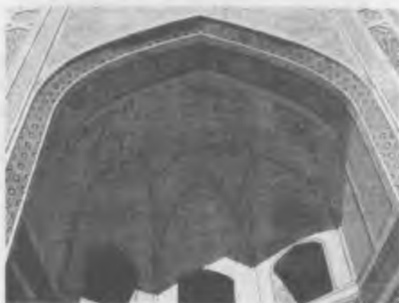
10.27-rasm. Masjidi Kalon darvozaxonasi gumbazining tuzilishi
