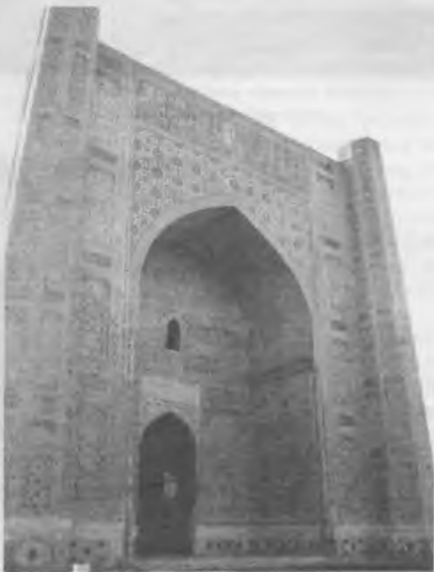
9.10-rasm. Masjid peshtoqining restavratsiyadan keyingi holati
