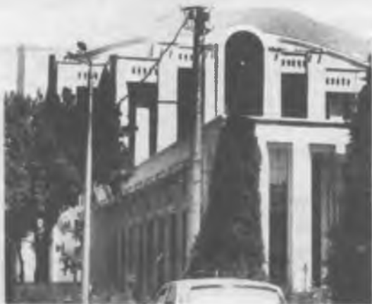
13.76-rasm. Toshkent shahridagi biznes-markaz binosi (orqadagi baland bino)
