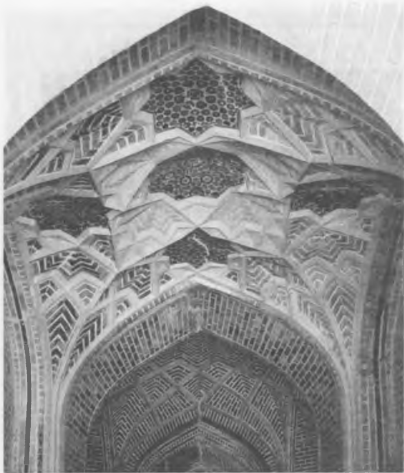
14.8-rasm. Turli materiallarga (ganch, sirli parchin va g'ishtga) naqsh solingan Nodir Devonbegi madrasasining darvozaxonasi gumbazi
