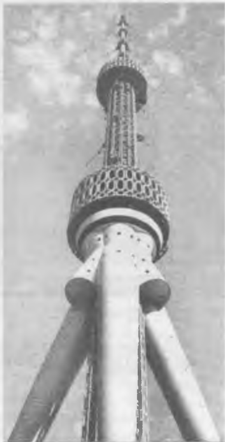
12.13-rasm. Toshkent shahridagi teleminora (1978–1985-yillar)
