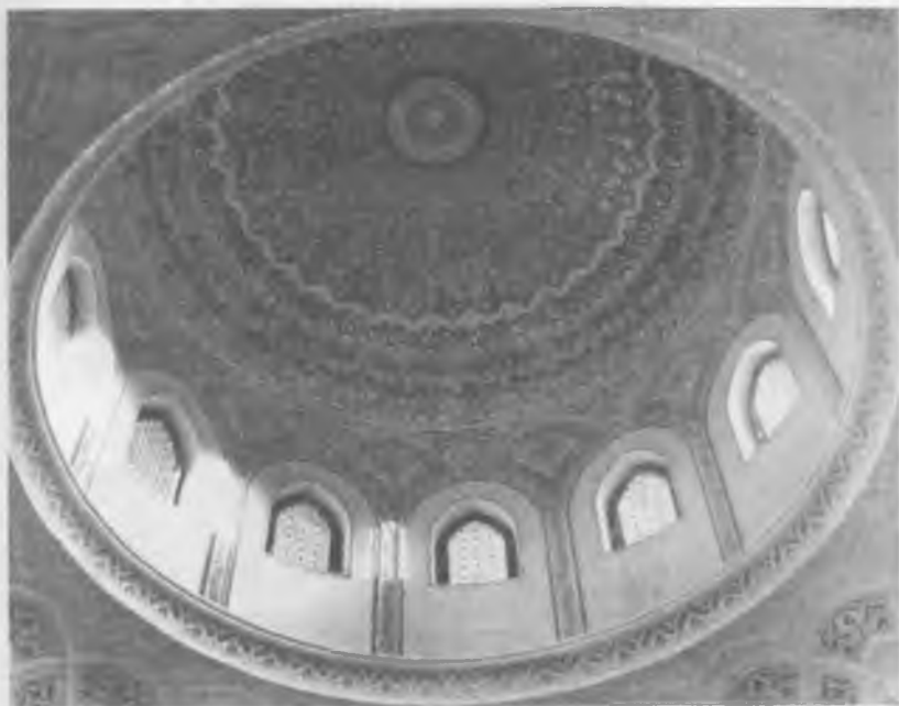
13.20-rasm. Milliy uslubda baraban shaklida bajarilgan provomli gumbazning ichki ko'rinishi
