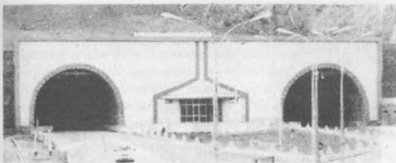
13.8-rasm. Qamchiq dovonidagi tunellarning kirish joyi
