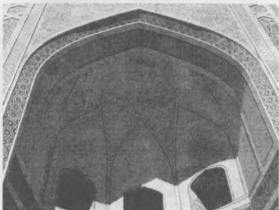
10.27-rasm. Masjidi Kalon darvozaxonasi gumbazining tuzilishi
