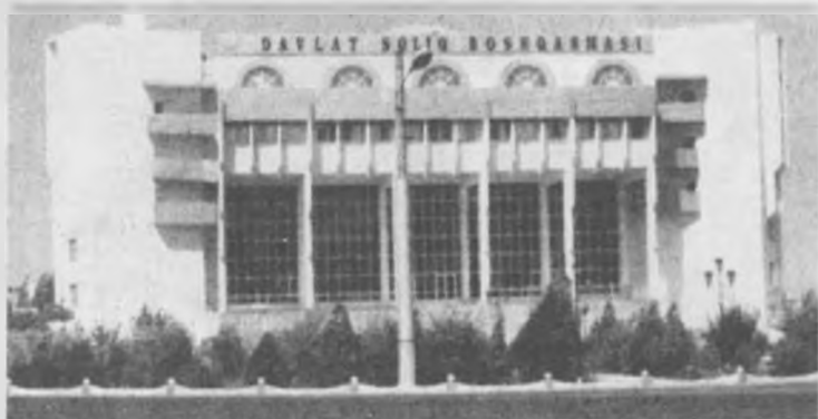
13.87-rasm. Urganch shahridagi soliq inspeksiyasi binosining ko'cha tomondagi fasadi
