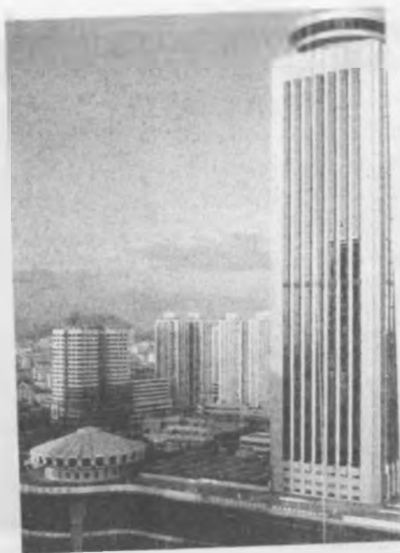
7.39-rasm Shanxay shahridagi zamonaviy osmono'par binolar
