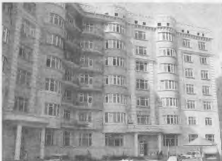
6.4-rasm. Toshkent shahridagi 7 qavatli zamonaviy turar-joy binosi
