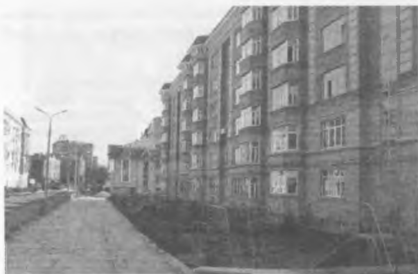
6.6-rasm. Toshkent shahridagi 6 qavatli zamonaviy turar-joy binosi
