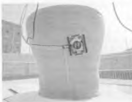
2.2.10-rasm. 3D-printerda qurilish inshootlarini yasash
