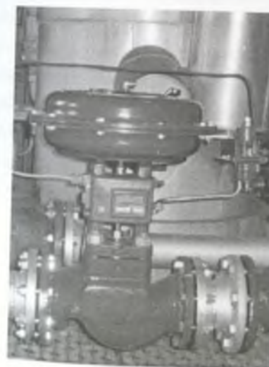
3.2.24-rasm. Rostlanadigan klapandagi membranali pnevmatik yuritma
