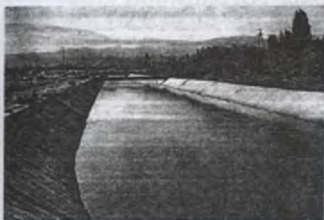
59-rasm. Yaxlit beton to'shamali kanal.
