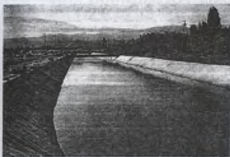
59-rasm. Yaxlit beton to'shamali kanal.
