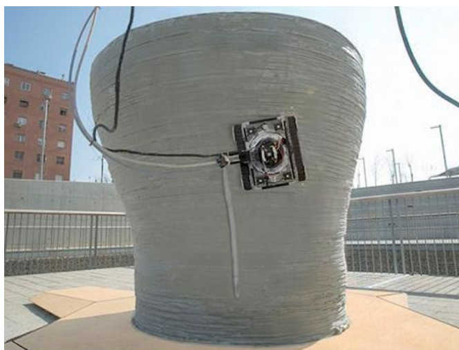
5.13-rasm. 3D-printerda qurilish inshootlarini yasash
