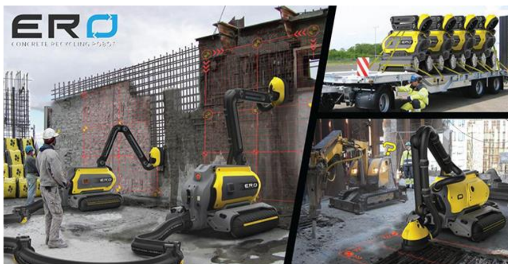
5.10-rasm. Robot demontaj ishini bajaryapti
