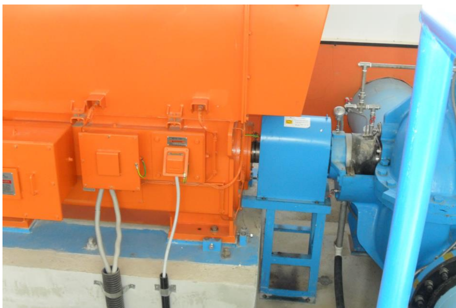
18.5 - rasm. Kabel liniyalarining elektr dvigatelga ulanishi
