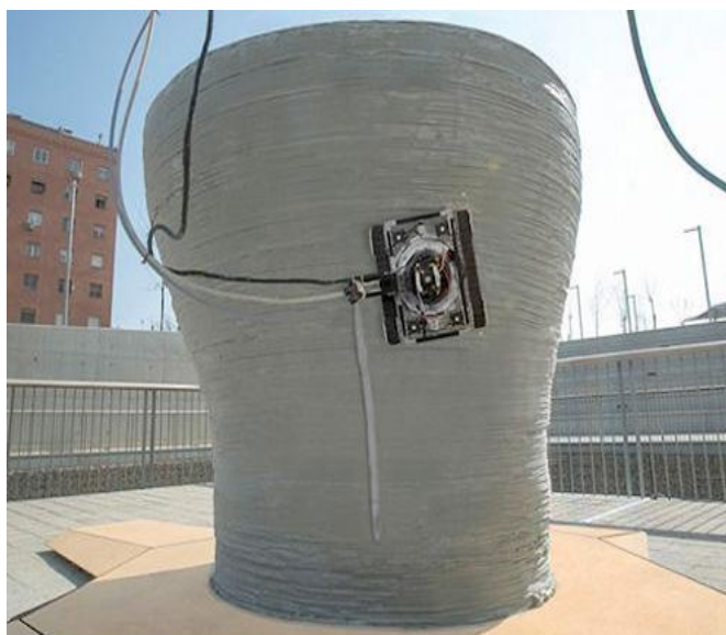
2.2.10-rasm. 3D-printerda qurilish inshootlarini yasash
