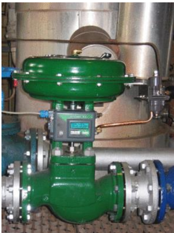
3.2.24-rasm. Rostlanadigan klapandagi membranali pnevmatik yuritma
