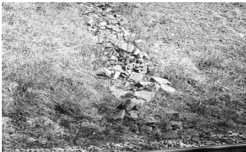
5.1-rasm. grunt qatlamining buzulishi.
