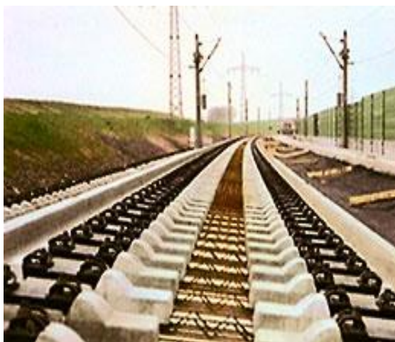
7.23-rasm. THM yo‘lining ustki tuzilishi:
