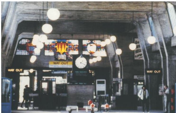
3.5-rasm. Temirbeton stansiya tomli Portal rama
