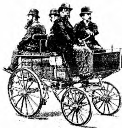
Fig. 2. Immisch&Company's electrified "dog cart"*
