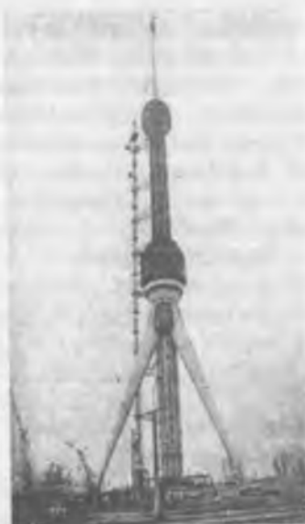
19.7-rasm. Toshkent shahridagi 350m.li teleminora.
