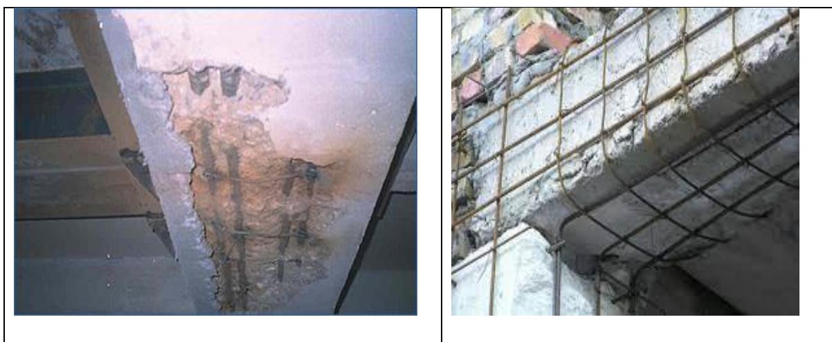
17.29-rasm. Rigelda armaturaning himoya qatlamini tushib, armaturaning zanglagan holati (a). SHikastlangan temirbeton rigelni temirbeton ko'ylak bilan kuchaytirish uchun armaturalangan holati (b).
