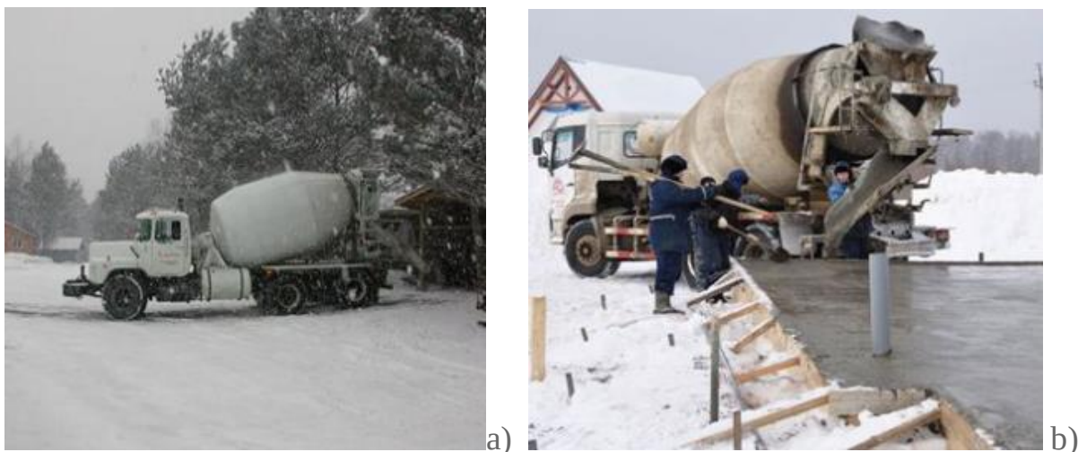
15.29-rasm. Qishda beton qorishmasini mikserlarda tashish (a) va poydevorga quyish (b).
