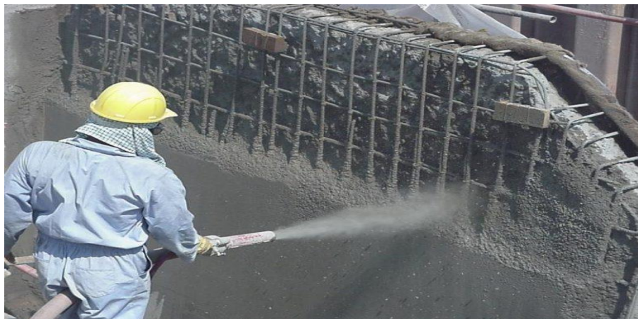
15.55-rasm. Torkret qatlamni to'shash jarayoni
