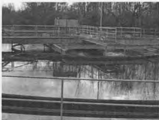
77-rasm. Ikkilamchi tindirgich.
