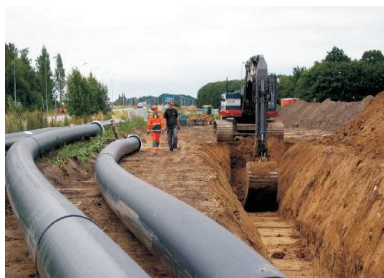
Figure 2 Poly(ethene) is used to make large water pipes
