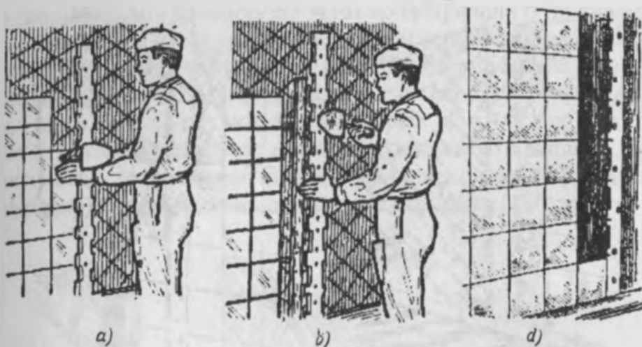
174-rasm. Afonin andazasi yordamida tik qator plitalarni terish: a) navbaidagi tik qatorni terish; b) o'lchov asbobi yordamida andazani o'rnatish; d) bir tomonlama andazadan foydalanish.
