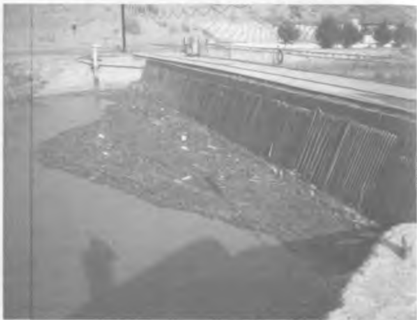
8.8 - rasm. Qo'qim ushlovchi panjaralar
