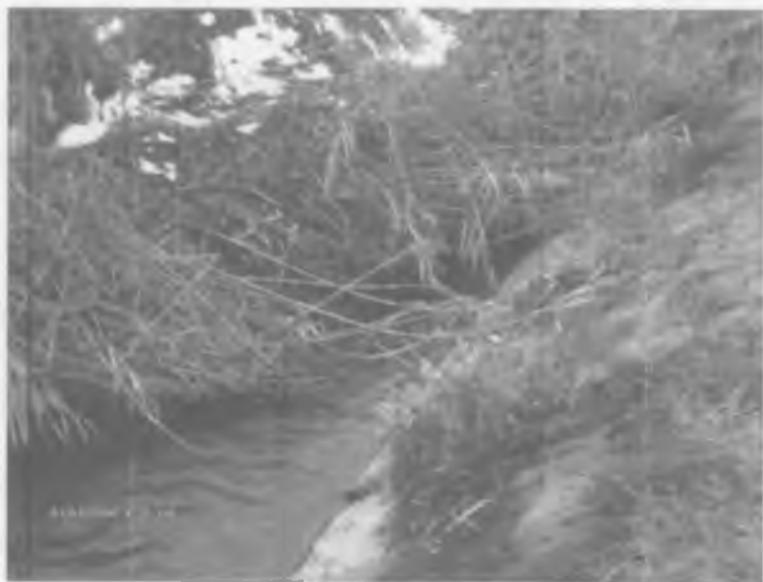
5.8 - rasm. Beton kanallar chetini o't bosishi
