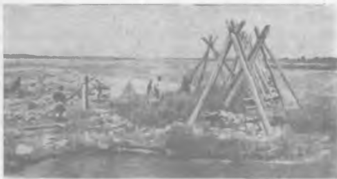
1.8 - rasm. Daryo o'zaniga sepoya o'rnatish.
