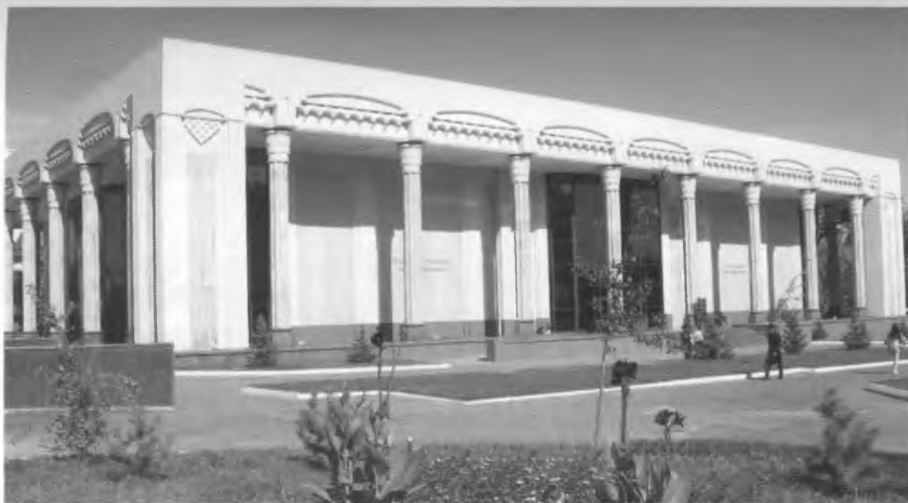
Toshkent. Tasviriy san'at galereyasi
